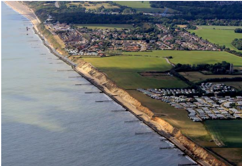
Aerial view of Corton and showing cliffs, groynes and caravan parks
